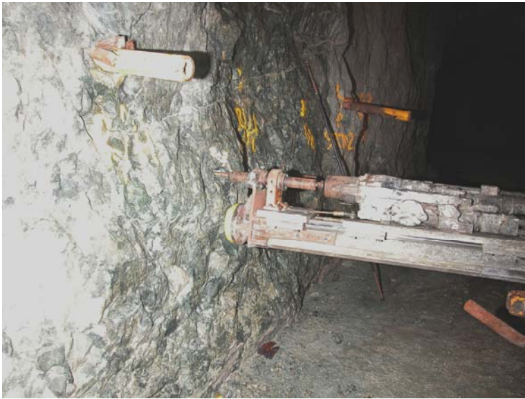
Figure 16: Trial bolt installation below simulated boreholes
