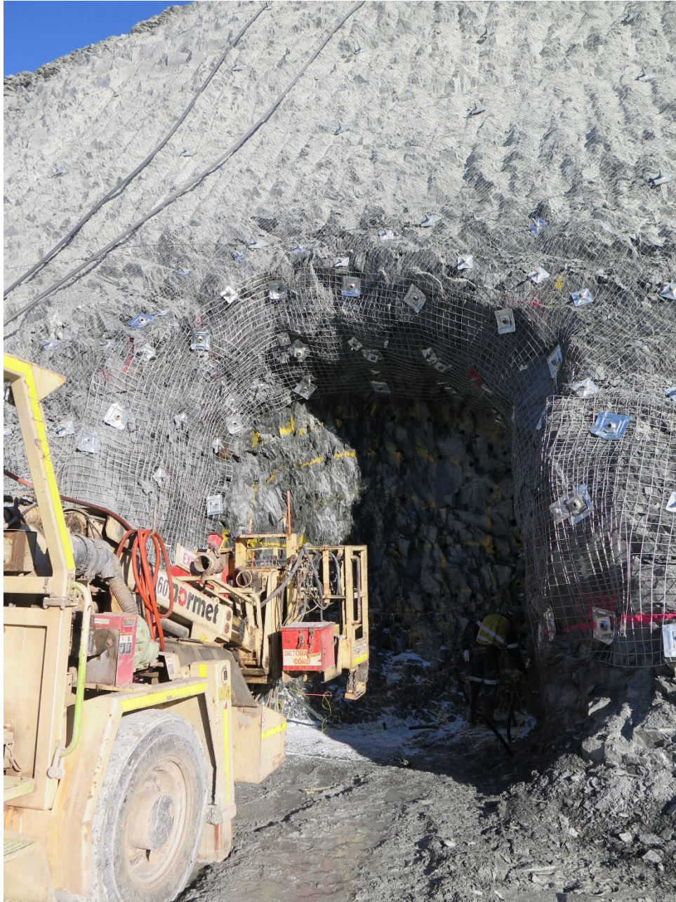
FIG 16 - Southern portal after blasting the first full cut.
