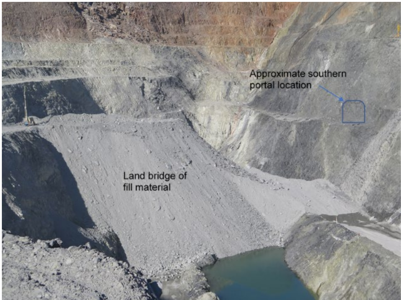
FIG 11 – Construction of land bridge for access to southern portal
