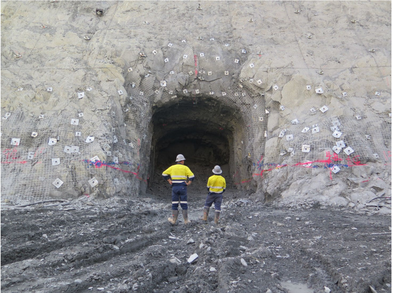
FIG 15 - Northern portal after mining first 4 cuts.
