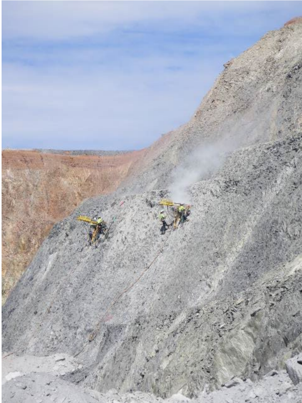
FIG 14 – Drilling of anchors using drills lowered from pit crest.
